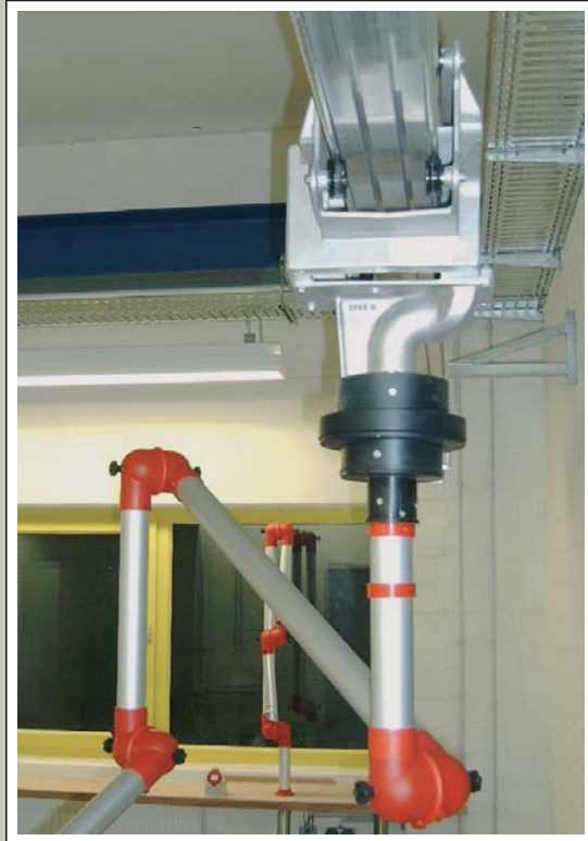
High vacuum system with SSK 50 and mini arm 50ø for polishing and grinding work places of long parts in the industrial processing of high integrated steel.
