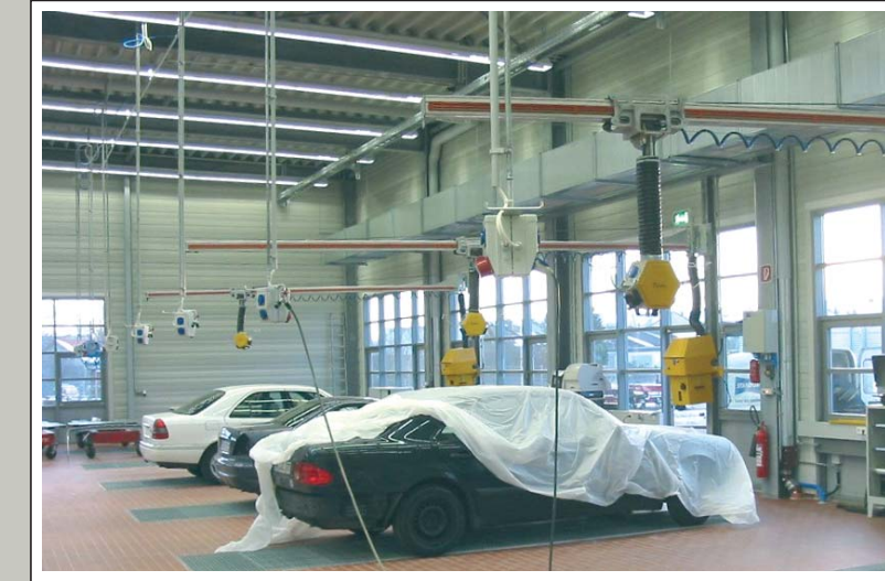
High Vacuum dust extraction system for paint preparing with aluminium rail system type SSK 50 - 6 m long, swivelling over 2 work bases. Each rail includes 1 trolley with an Energy box (2 dust suction points, 2 electric connections, 2 compressed air connections).
