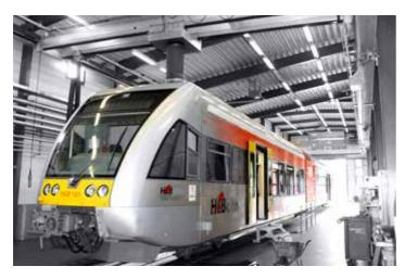
**Movable extraction racks** – The electrically-driven extraction racks are ideal for use on larger extraction areas over several rails. Our wealth of experience means that we can find a solution for any problem regarding the capture of harmful substances from diesel engine emissions.
