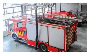
exhaust gases. This leads to a much lower load on the suction hose and extends their useful life.
