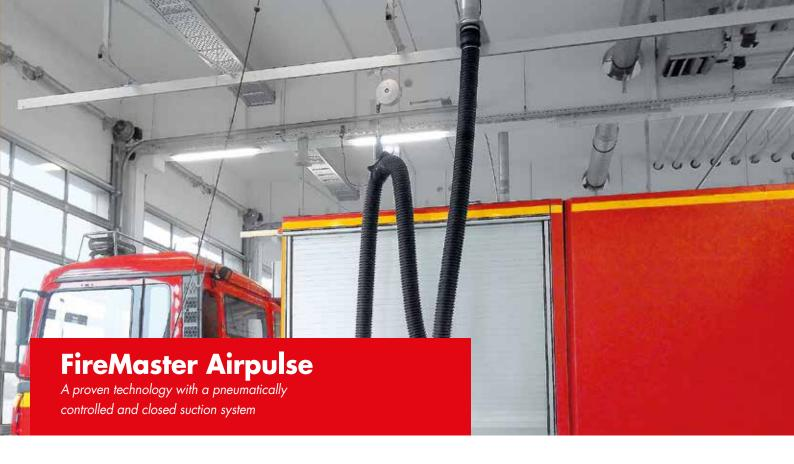
The **s.tec Germany** FireMaster Airpulse system is a pneumatically controlled, automatic exhaust gas extraction system. This system was developed especially for emergency vehicles with side, rear, or bottom tailpipes. The exhaust gases arising are recognised directly at the exit point. A pneumatically operated collar causes the frictional sealing of the exhaust and thus extracts the exhaust gases.
