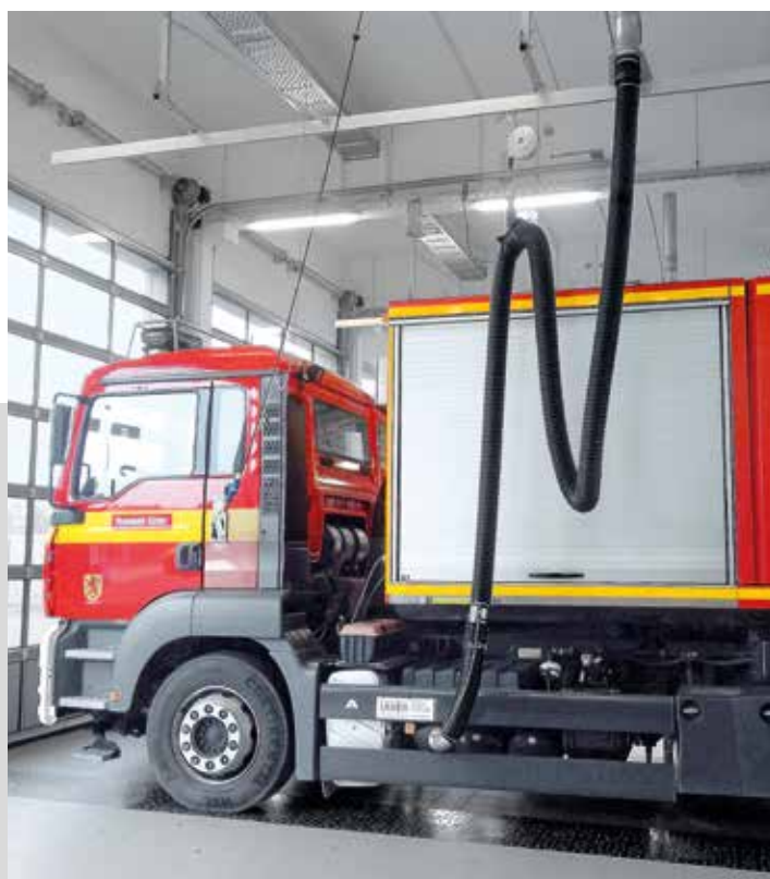
Ceiling guidance near the vehicle ensures freedom of movement.
