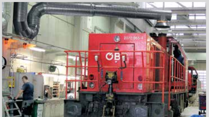
Diesel locomotive-extraction with pivoting side arm.
