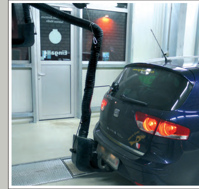
Capture element from Type "SLS-Car" in modified form for travelling along over the controlling track.
