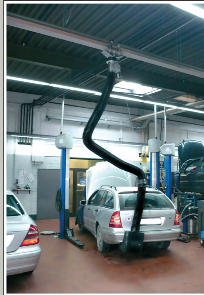
SLS Car-AU with a DN 150 hose for the gas emission tests. There is no need for the common separate standing funnel any more.
