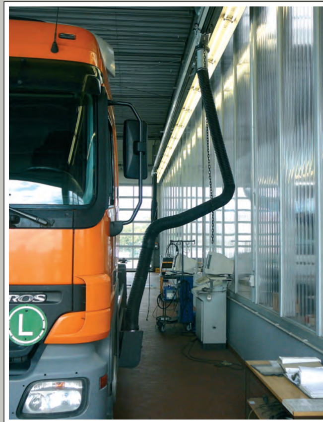
"SLS-Truck" for automatic travel-along and gas extraction of trucks over a brake tester at a Mercedes-Benz truck workshop.
