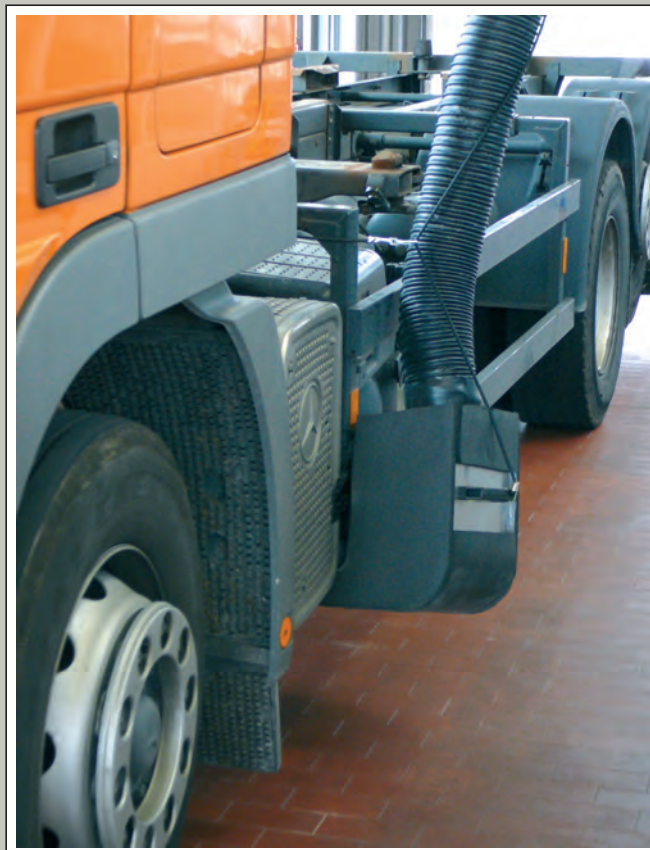
"SLS-Truck" for automatic travel-along and gas extraction of trucks over a brake tester at a Mercedes-Benz truck workshop.
