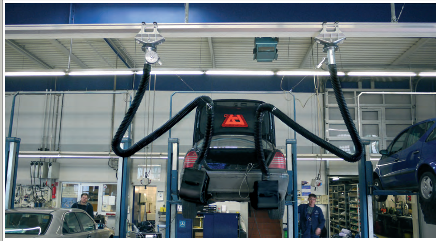
2 SLS – Car systems running in a suction rail from type SSK 150150 by the automatic travel-along for works on the lift with a running engine.
