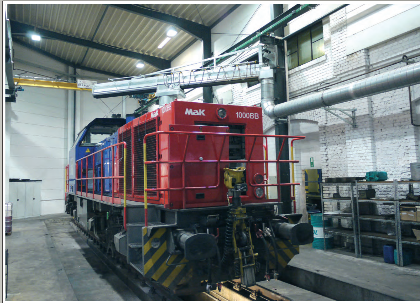
Diesel locomotive extraction in a Vossloh-Werke service workshop with a swivel-mounted SSK 900 rail system for up to 10,000 m 3 /h, adjustable in three axes.
