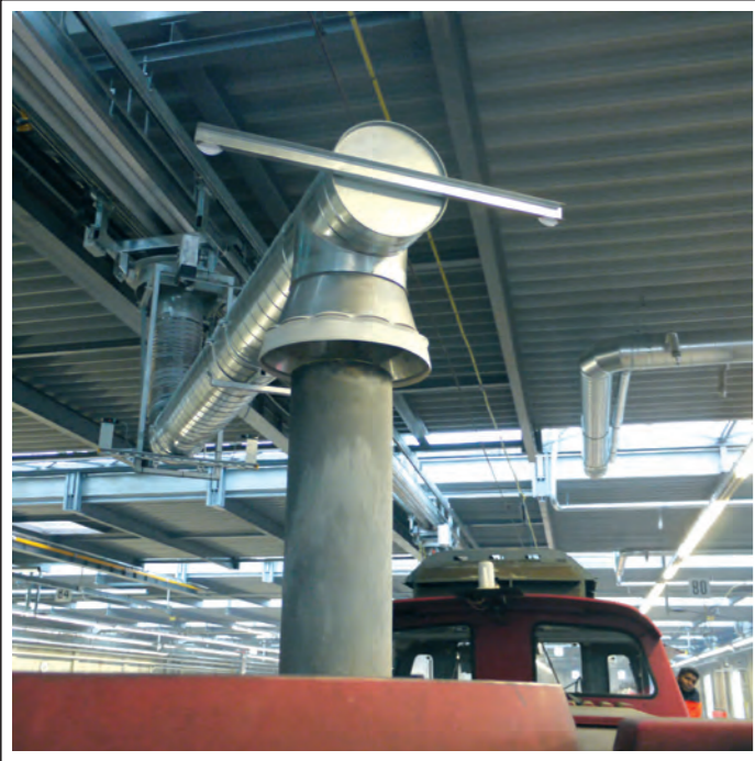
Extraction cover NW 550, height adjustable with extraction arm NW 355, swivelled below a catenary wire with mixed operation of diesel and electric locomotives.
