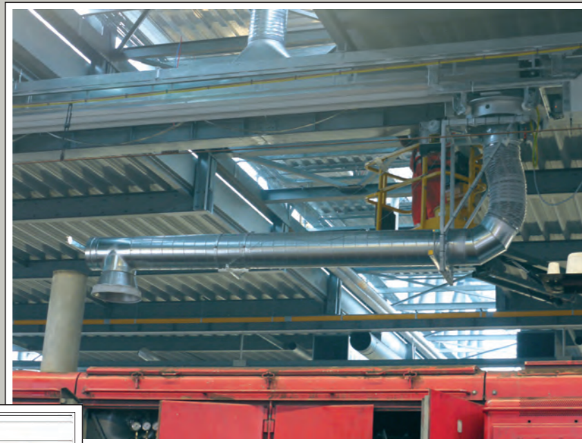
Extraction arm NW 355, movable in three levels in an SSK 900 rail system across a length of 50 m, with radio remote control.
