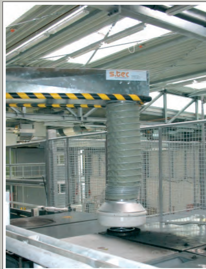
Telescopic extraction cover for a diesel railcar.
