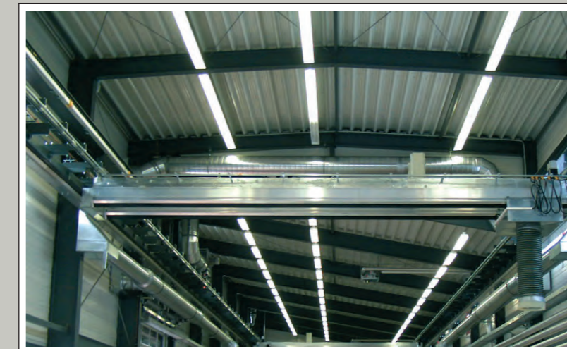
Diesel locomotive extraction with extraction rack and telescopic extraction cover – 2 m – in NW 355 for 6,000 m 3 /h.
