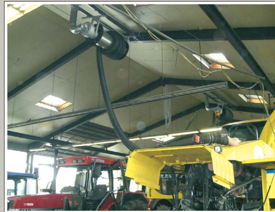
Compact hose reel with fan mounted on the side. Hose length: 15 m.
