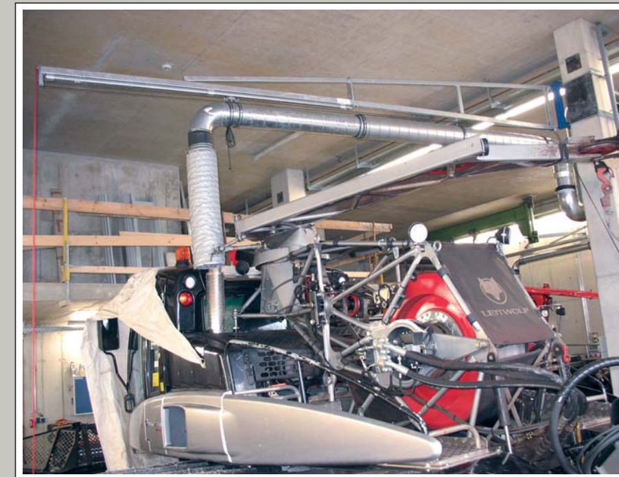
Telescope pipe boom in high temperature version for special vehicles.
