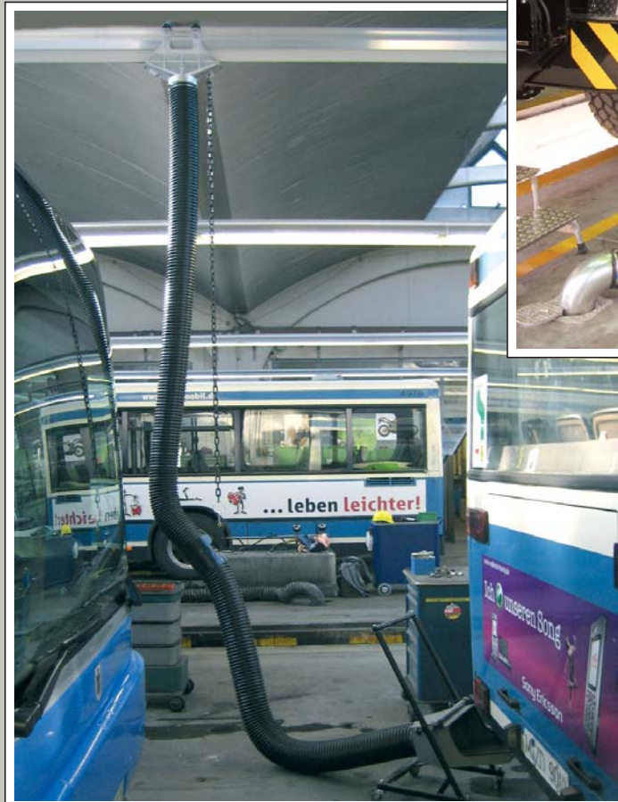
Mobile extraction hose reel (on carriage) for overhead high exhaust systems. Easy attachment on existing under floor extraction system.
