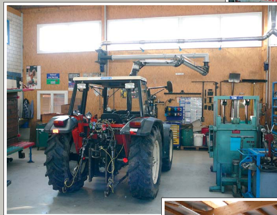
Extraction arm with a reach of 8 m for upward facing exhaust pipes
