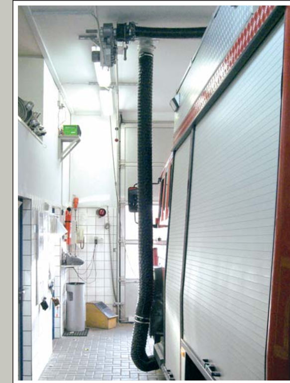
FireMaster Start For smaller fire brigades with a low usage rate where no riding-along system is required. The FireMaster Start hangs freely without a foot stand. Thus no tripping hazard. Only for the starting procedure, is subsequently removed without problems from the vehicle after driving off.
