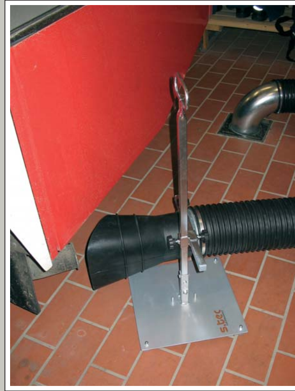
FireMaster Ground Underfloor system with underground extraction pipes and short hoses with exhaust extractors. This reduces the tripping hazard and the equipment can be cleared away quickly and completely, if required, to make room in the fire brigade hall.
