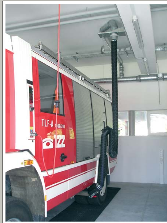
FireMaster Classic A tried and tested system, if you only need to cover a short distance from the parking position. This is the case, if the exhaust is installed very far forward on the vehicle. No rails or the like are necessary here.
