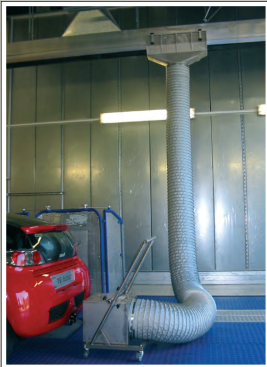
Exhaust extraction system for Dyno tests, designed for an engine power of maximum 1,000 kW. 2x Extraction rail system from type SSK 450 each equipped with exhaust extraction hose with temperature resistance till 850°C and special "down-slide" stainless steel funnel.
