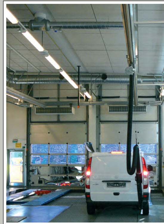
Exhaust extraction system specially designed for vehicle inspection stations with (TÜV, CT, CRV, NCT, ITV, APK, MOT, SWEDAC, etc...) equipped with 2x extraction rail system from type SSK 290 and return transfer station.
